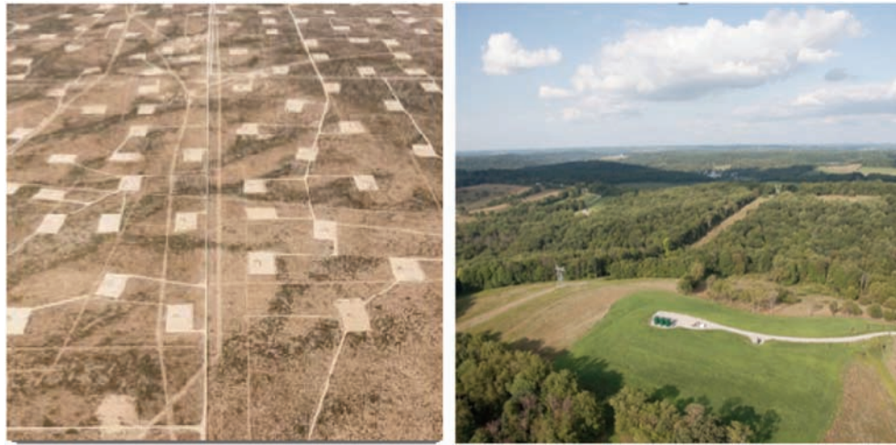
Figure 2 Innovation in well design and operation (source: Range Resources Ltd.). Left: old single well spacing (Texas); right: modern multi-well cluster configuration accessing gas from an area of up to 10 km 2 (Pennsylvania).
